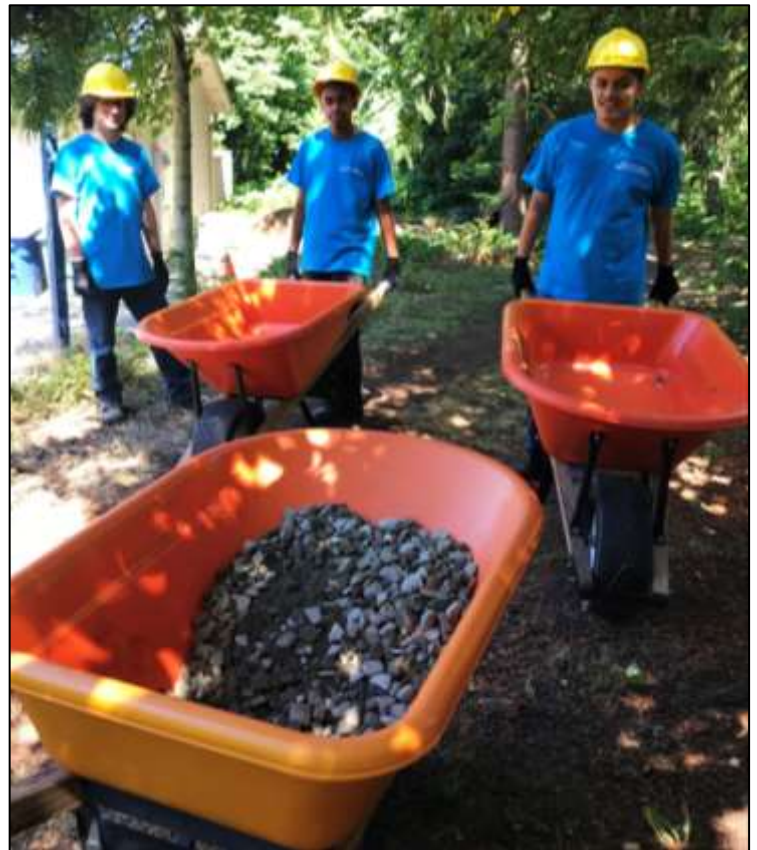
Trainees transported and spread gravel at Lower Coal Creek
